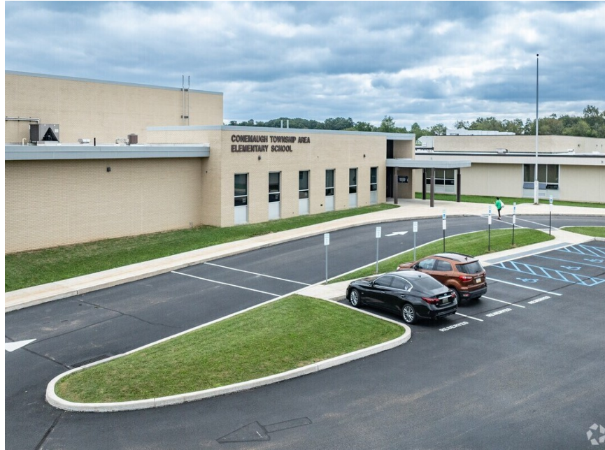
Photograph 1 —View of Conemaugh Township Elementary School located at 1516 Tire Hill Road, Johnstown PA.
