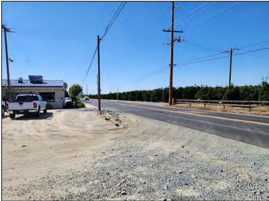
View 2: From the north side of the project site, looking northwest along West Teapot Dome Avenue and at agricultural uses and Hope ES buildings west of the project site.
