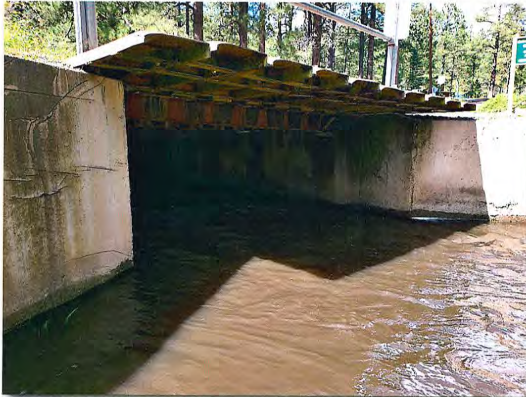
Photo 1. Elevation of existing bridge located on County Road 1009 near Greer, AZ.
