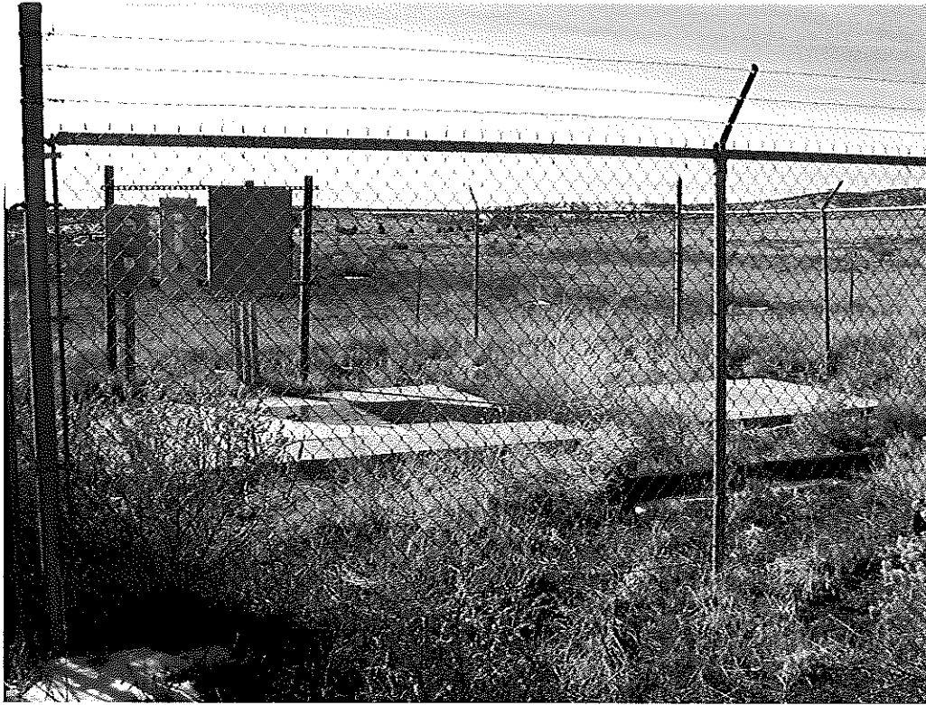
Figure 17. Exterior of Main Lift Station
