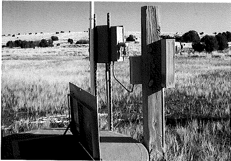
Figure 2. Exterior of Lift Station 9A
