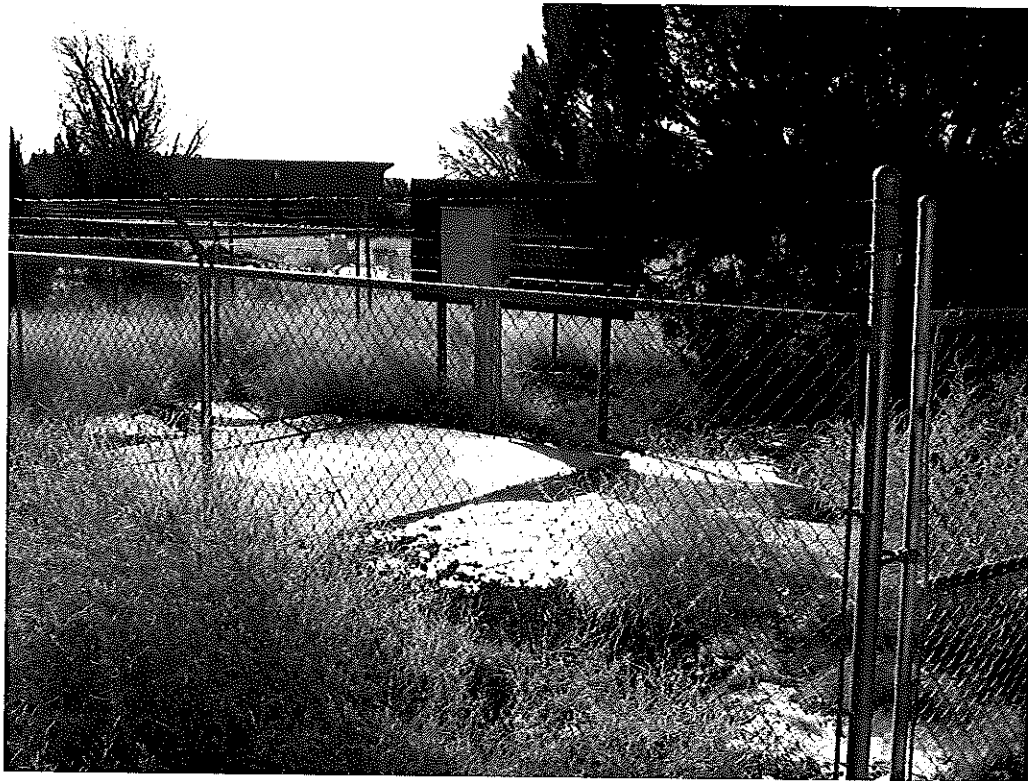
Figure 11. Exterior of Golf Course Lift Station
