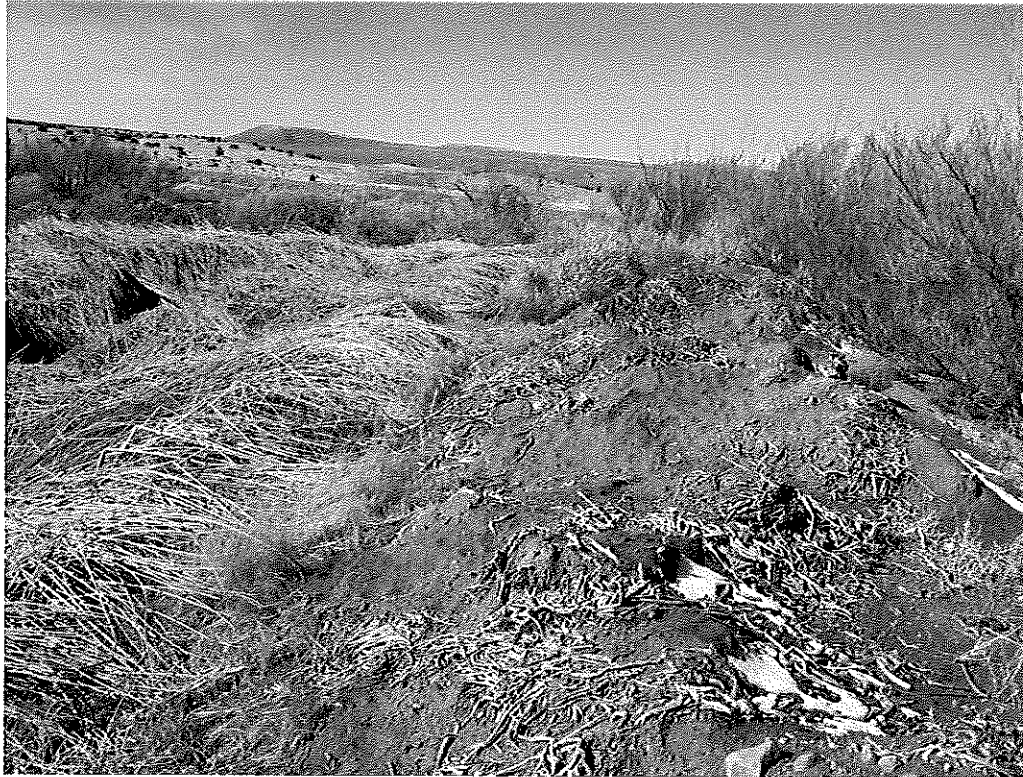
Figure 24. Settling Pond Berm
