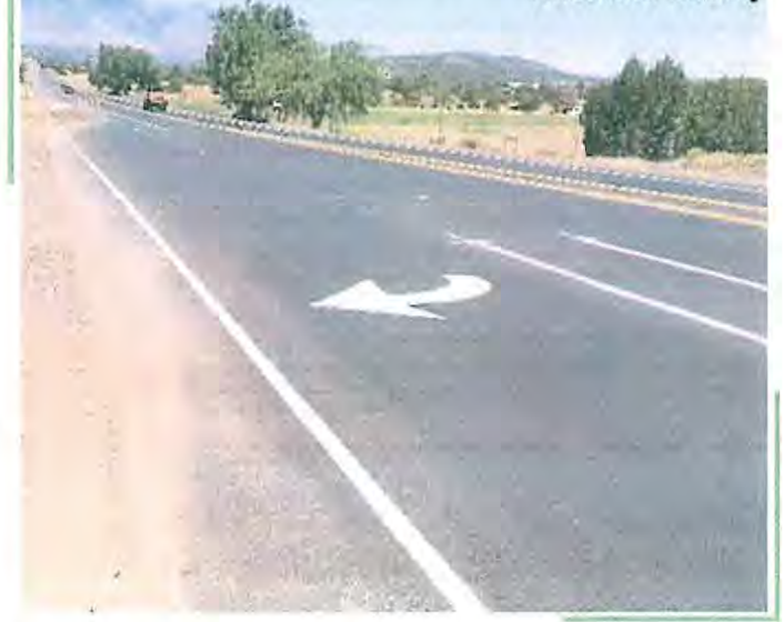
Townsend-Winona Road Pavement Rehabilitation Coconino County
