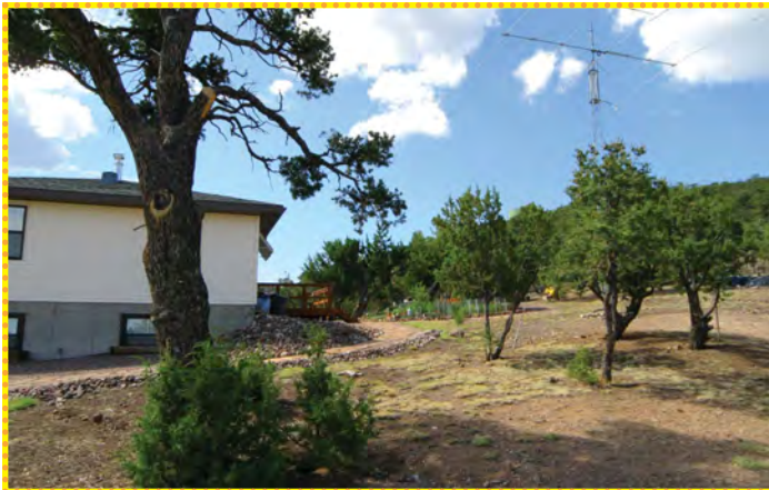
Treated Private residence using fire-safe techniques Source: Town of Eagar
