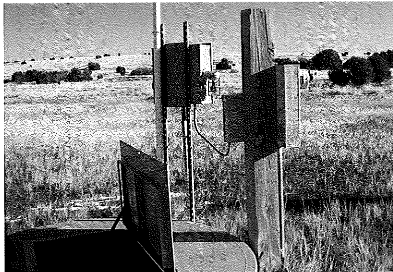
Figure 2. Exterior of Lift Station 9A
