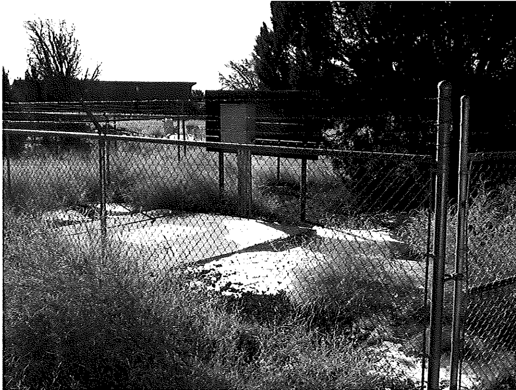
Figure 11. Exterior of Golf Course Lift Station
