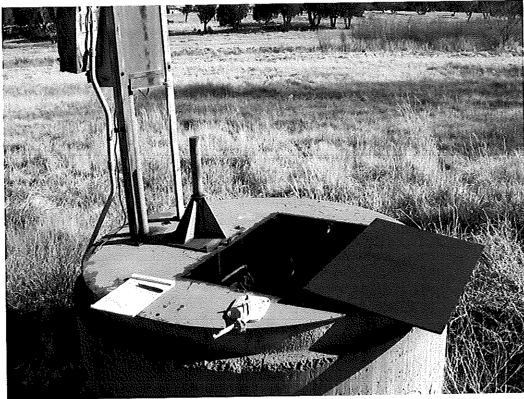
Figure 15. Exterior of Motel Lift Station
