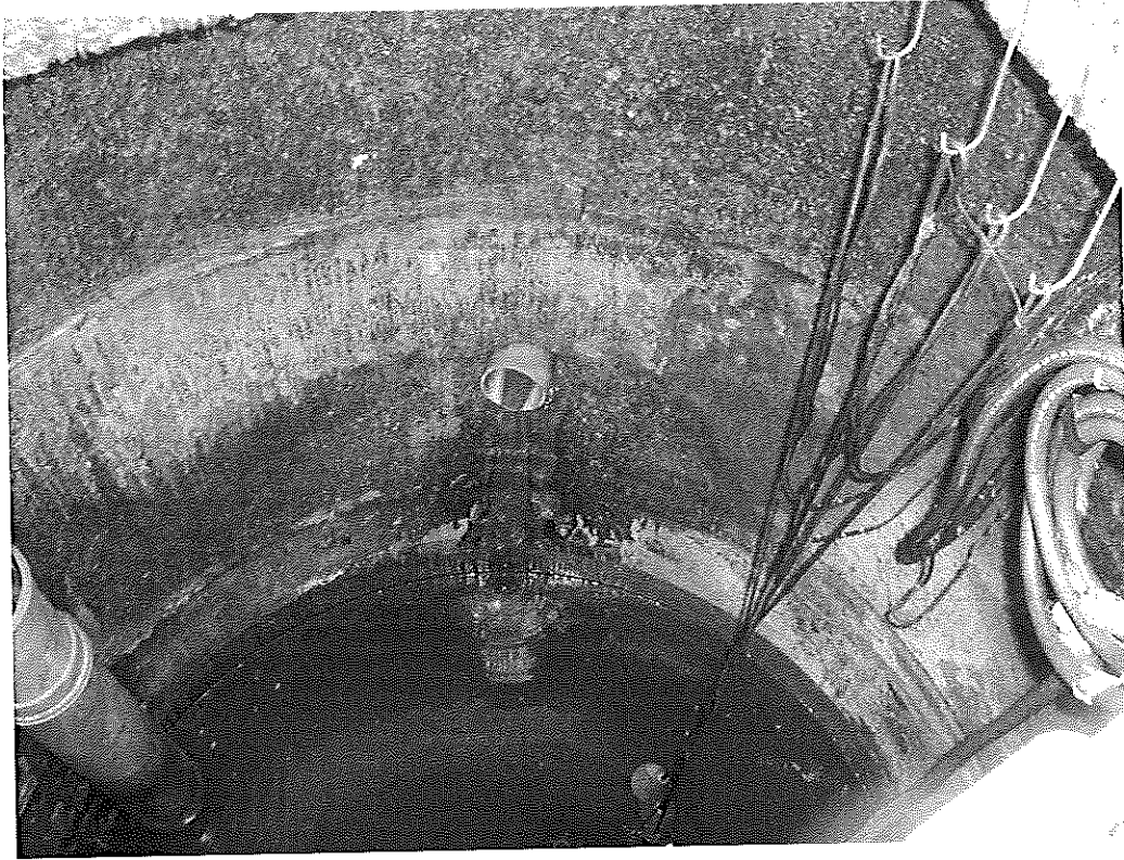
Figure 13. Interior of Golf Course Lift Station
