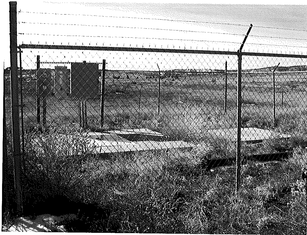
Figure 17. Exterior of Main Lift Station
