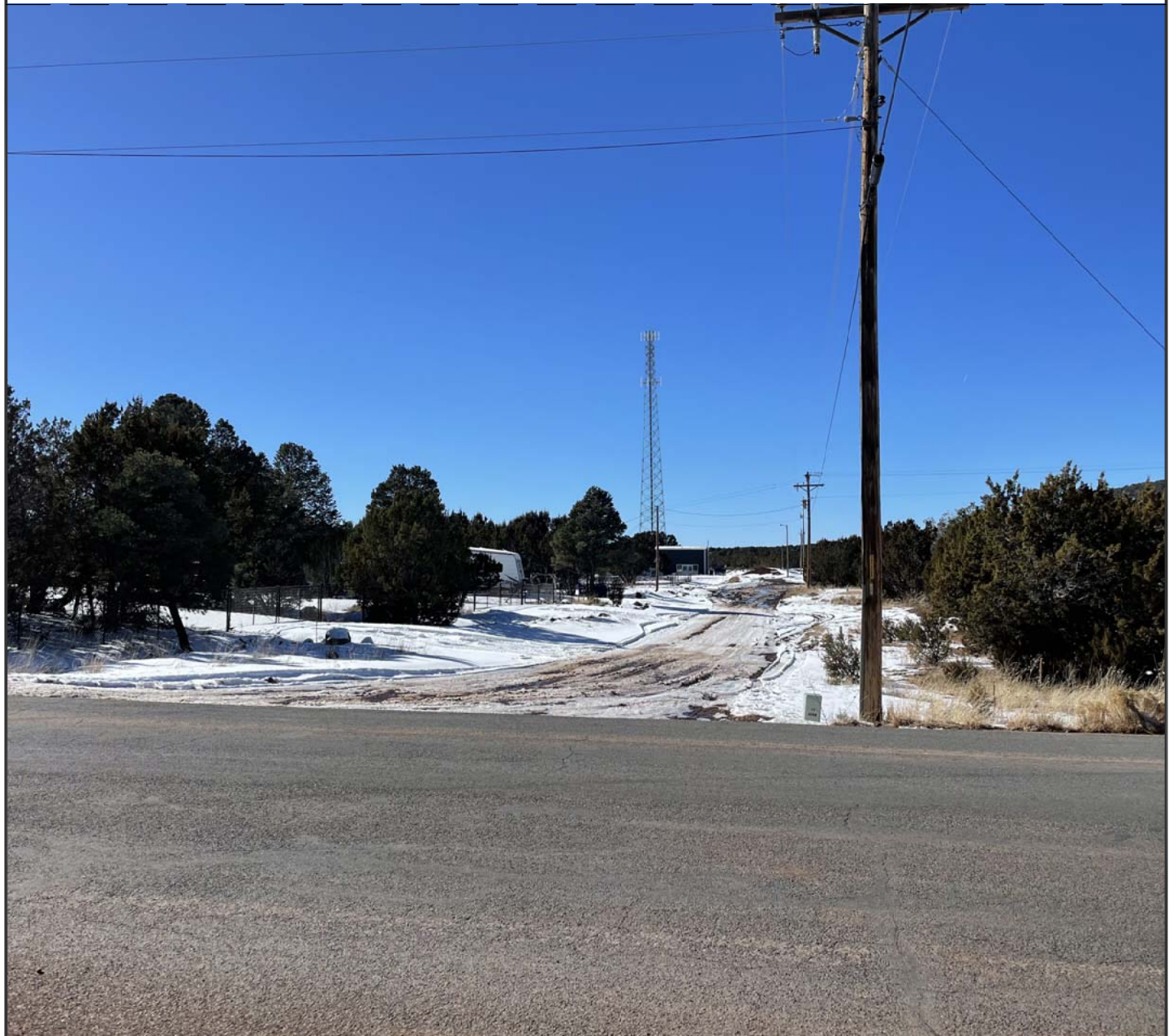
Looking West Toward Proposed Tower (After)
