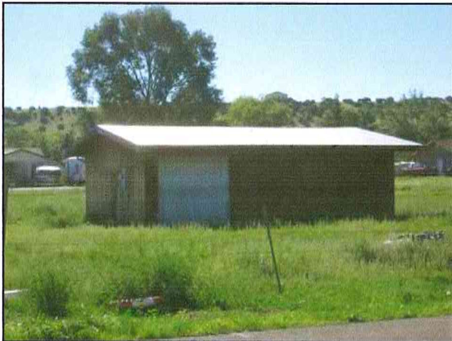
View of the existing building which encroaches on the subject parcel.
