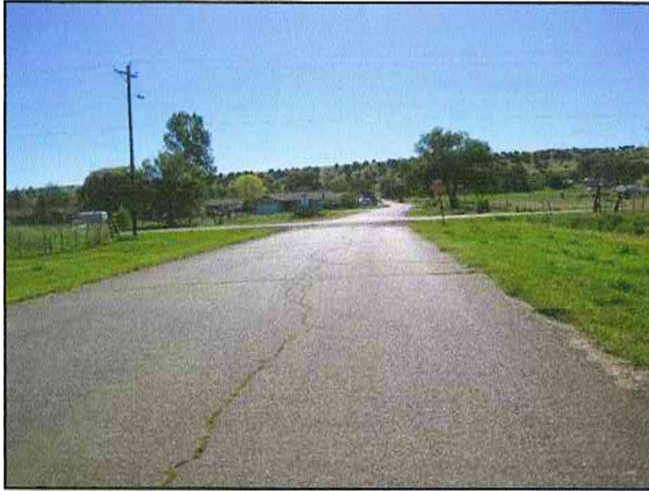
Street view looking east on 3 rd Avenue.
