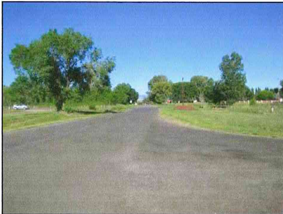
Street view looking west on 3 rd Avenue.
